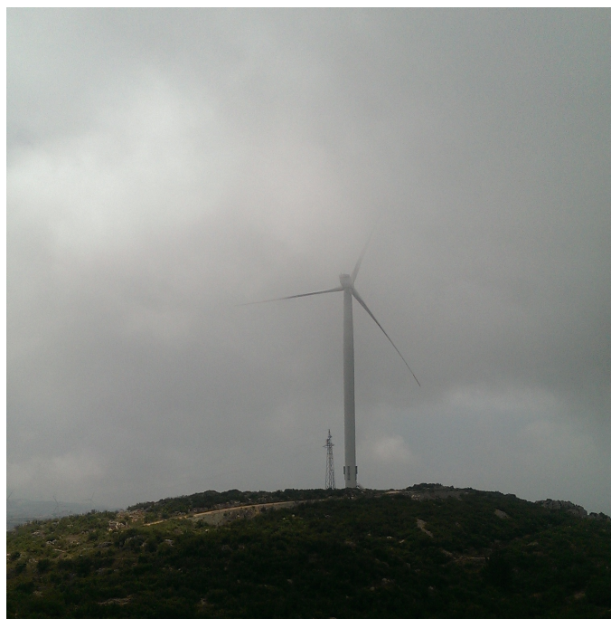
Figure 1: GE 2.5-100 wind turbine encounters fog in July, 2015, Samandağ, Turkey.
