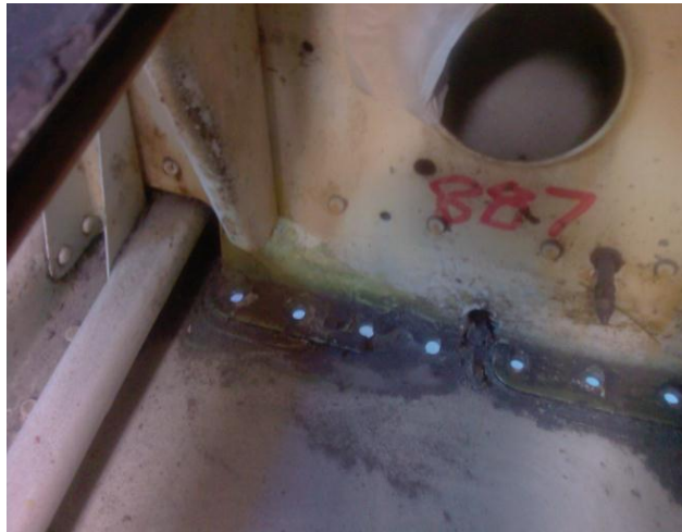
Figure 2: A View of the Corrosion in the Aft Cargo Compartment
