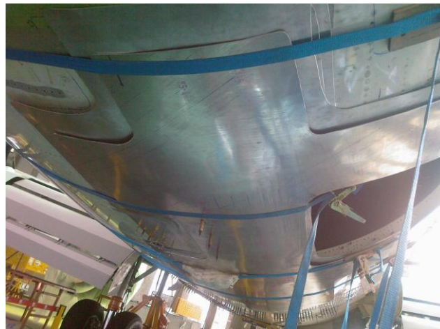
Figure 9: Fastening the Patches to the Fuselage of the A/C
